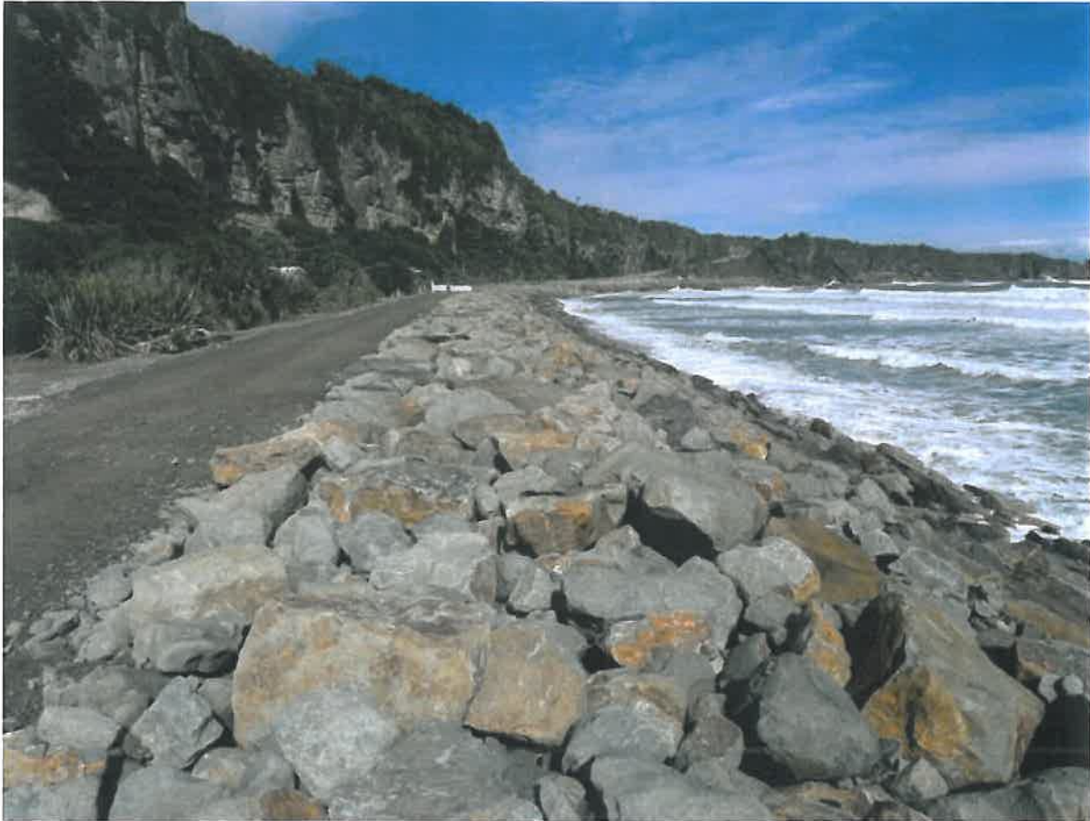
The completed Punakaiki seawall repair works
