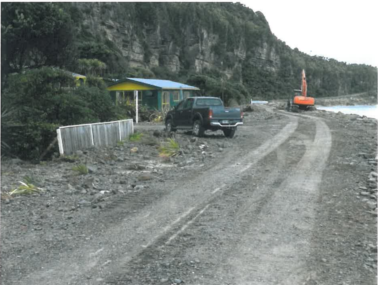
Damage to fences from recent high seas
